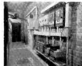
Layout of wall-mounted switchgear. Heavy components are installed at floor level which eliminates need for reinforcing the tile wall.
